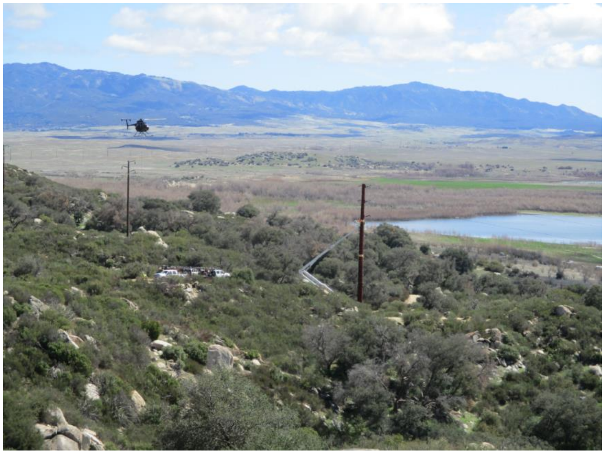
Photo 1: Preparation for wire stringing observed at Z118161 (TL 682).
